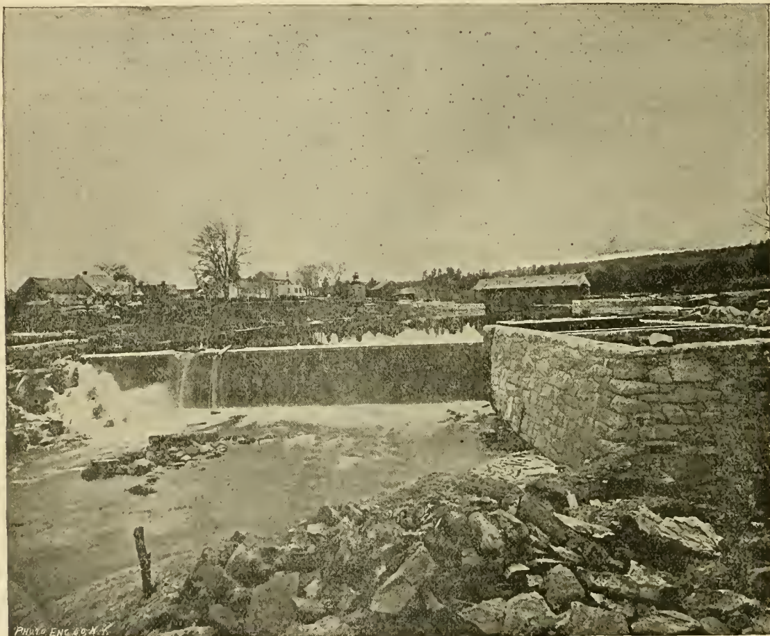
NEW DAM ON THE CONTOOOCK RIVER AT PENACOOK.
